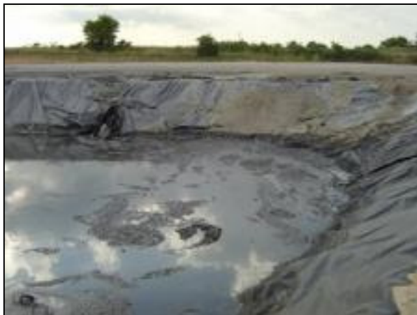
Waste pit near hydraulic fracturing job (Photo by TXsharon)
